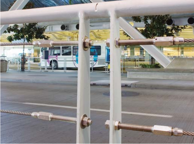
Stud Fitting - Lane Dividers and Safety Rails - Portland International Airport
