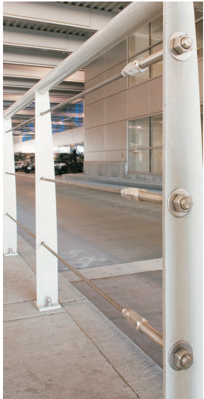
Stud Fitting - Pedestrian Walkway - Portland International Airport
