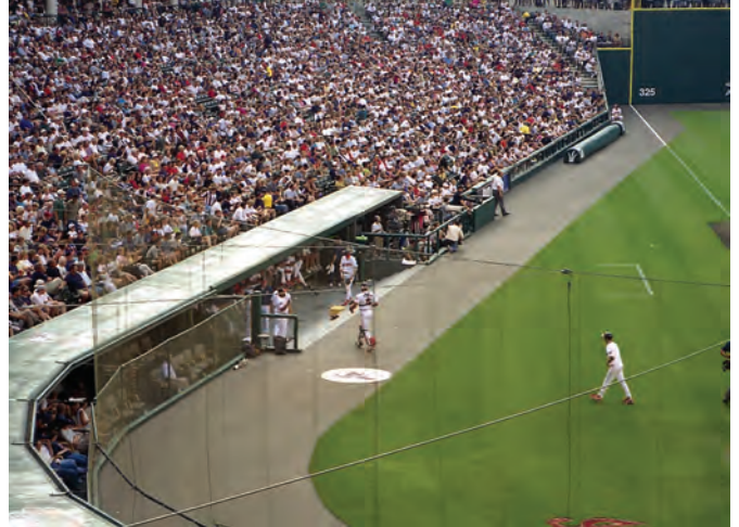
Clevis Fitting - Backstop Netting - Progressive Field - Cleveland, OH
